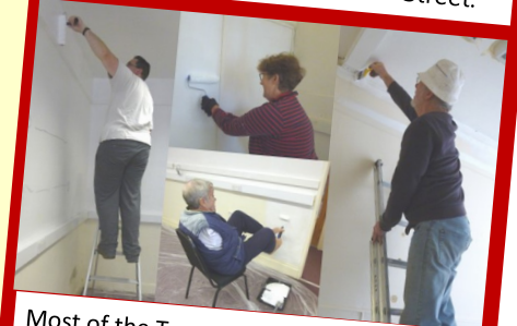
Most of the Town Council helped to paint the new offices.
